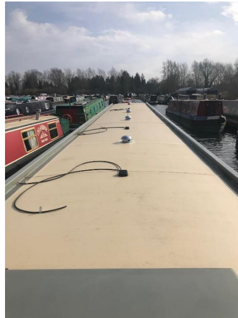
▲ Roof with 3 x solar panel to be fitted
